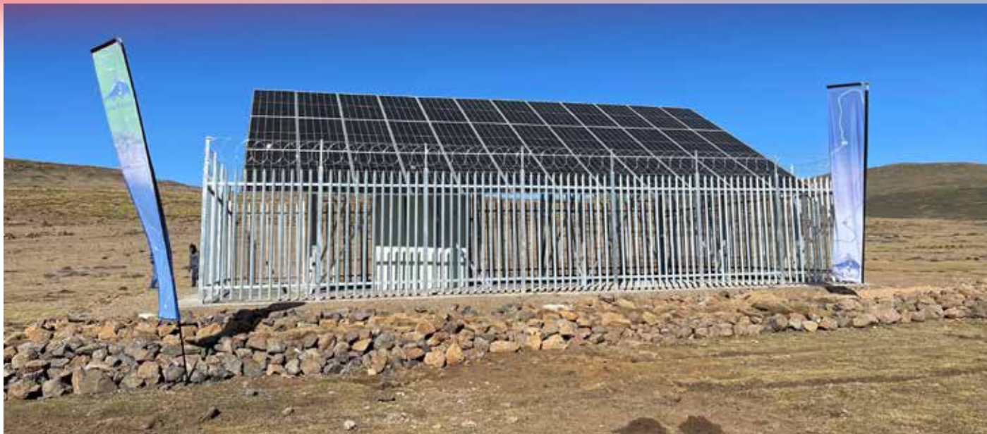
Solar Power Plant erected by Road Fund for Sani Border Post in Mokhotlong
