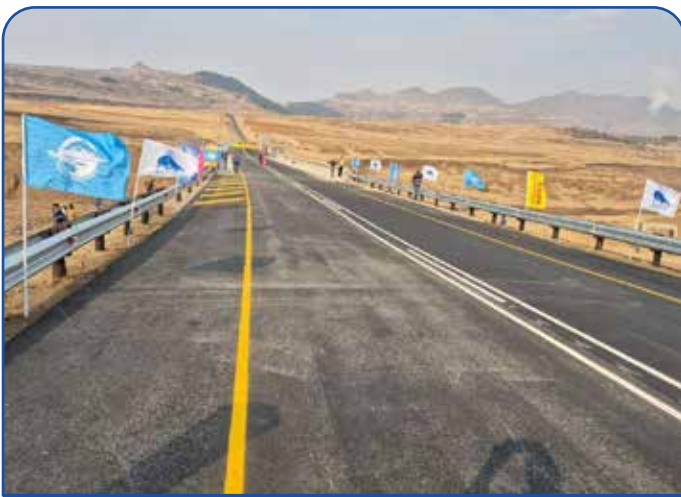
Branding of the Linoto Pholoana Memorial Bridge during its launch
