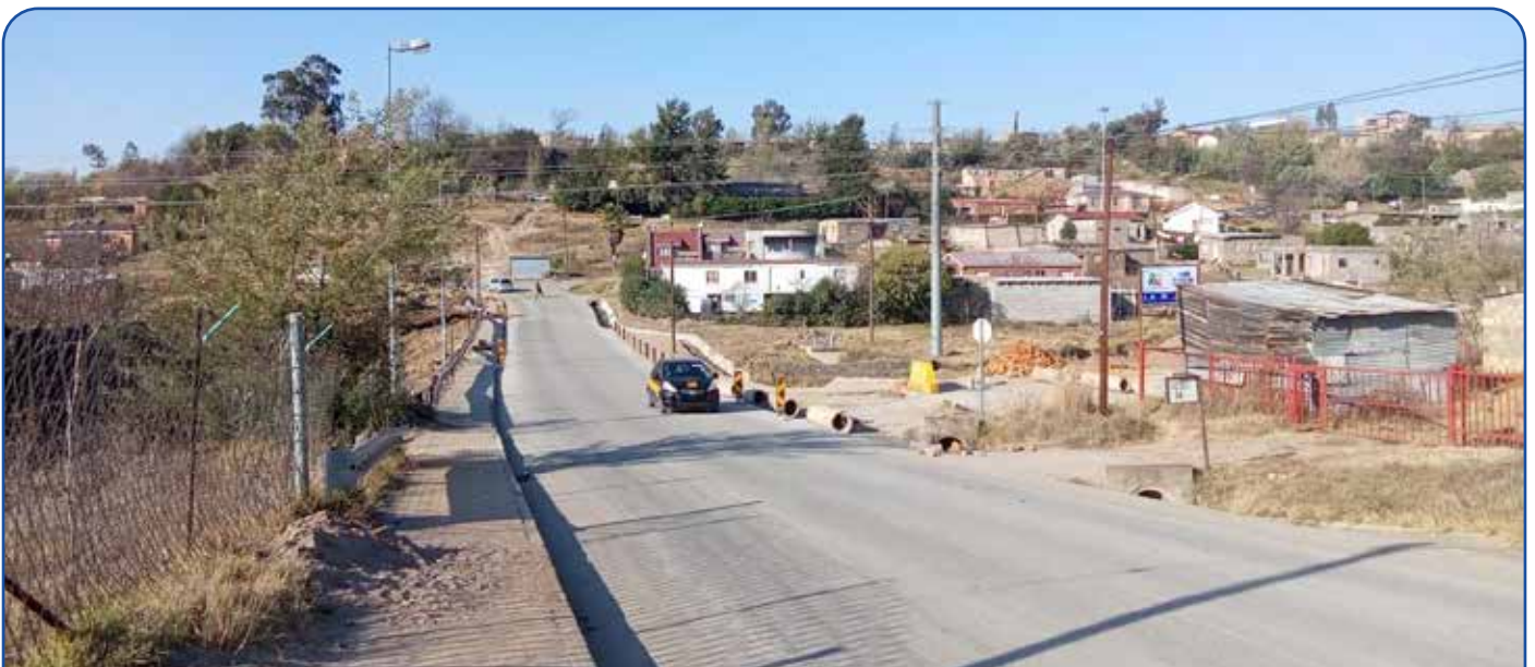
Periodic maintenance of C- Point to Moshoeshoe Airport Roads intersection and C point bypass
