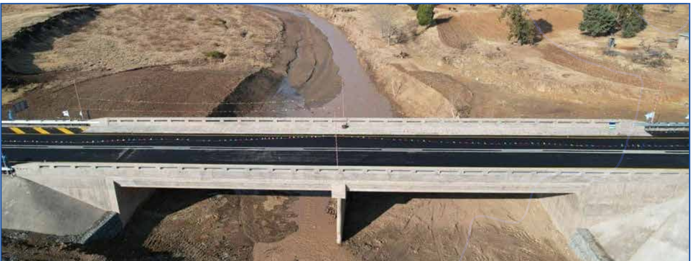
The newly constructed Linoto Pholoana Memorial Bridge
