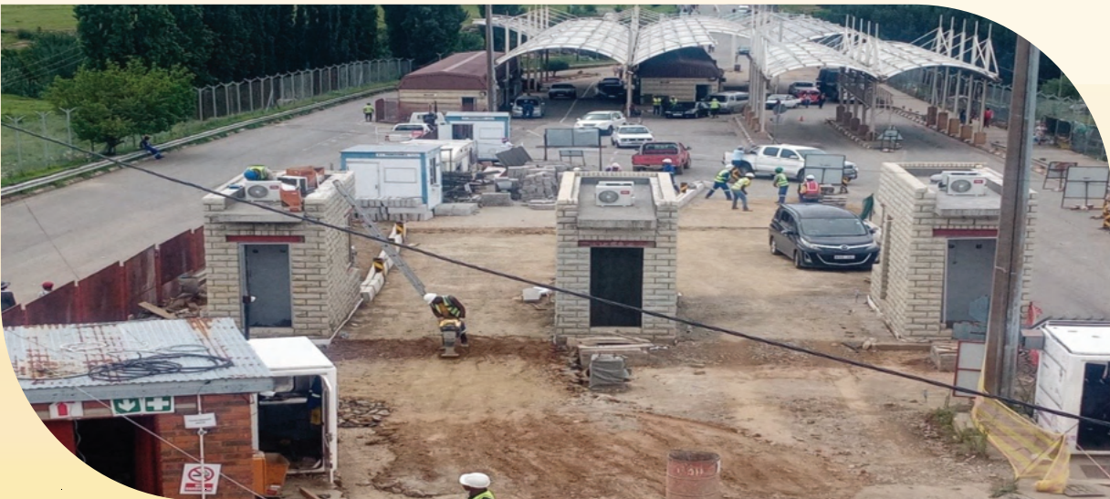
Pic 4: Construction of a Toll Facility at Maputsoe Border
