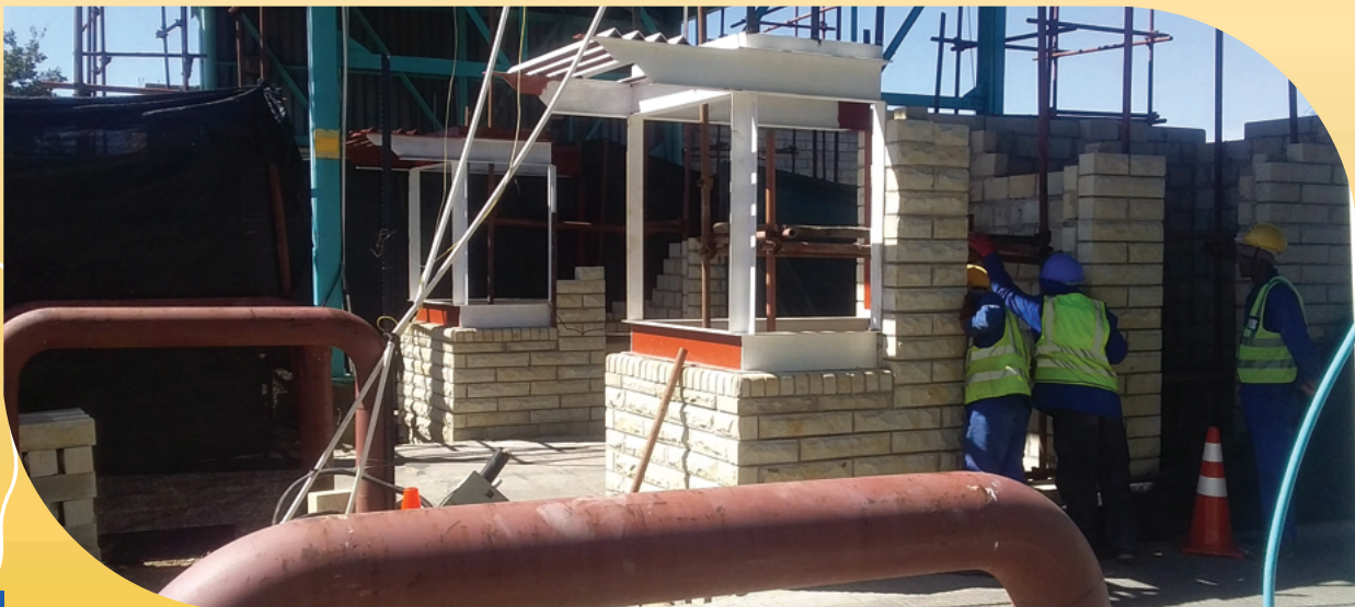
Pic 5: Construction of a Toll Facility in Maseru Bridge
