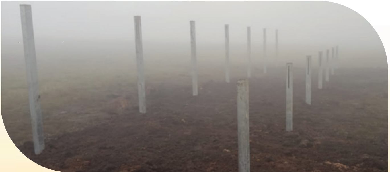
Pic 6: Solar array mounting structures erected
