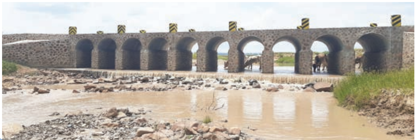
Routine Maintenance of Bongalla to Maoela Road - Construction of a Vented Ford
