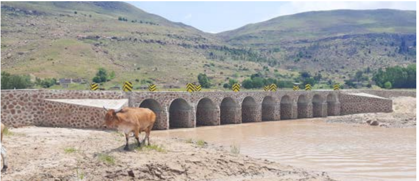
Routine Maintenance of Bongalla to Maoela Road- Construction of a Vented Ford
