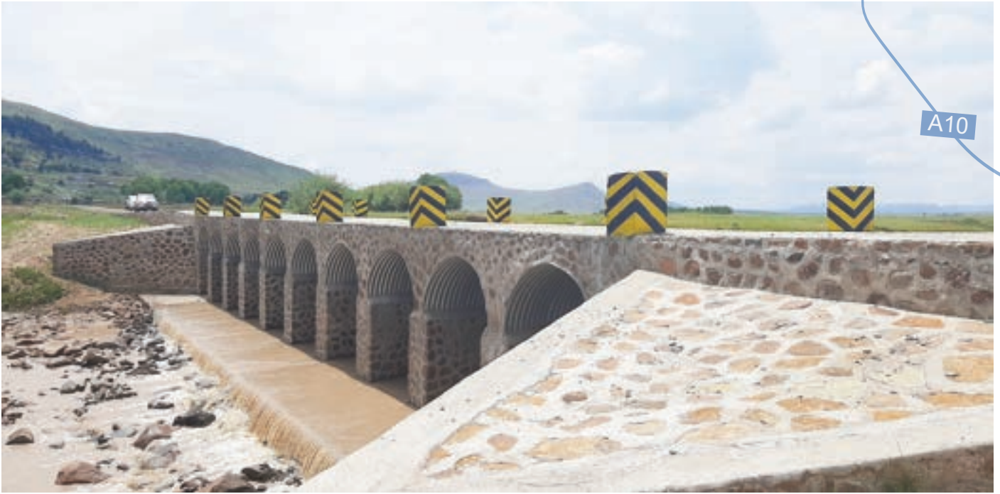
Routine Maintenance of Bongalla to Maoela Road- Construction of a Vented Ford
