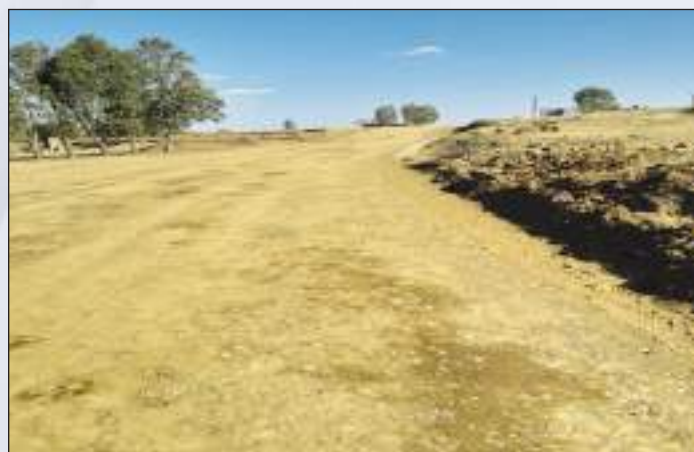
Tsakholo – Litšoeneng Gravel Road
