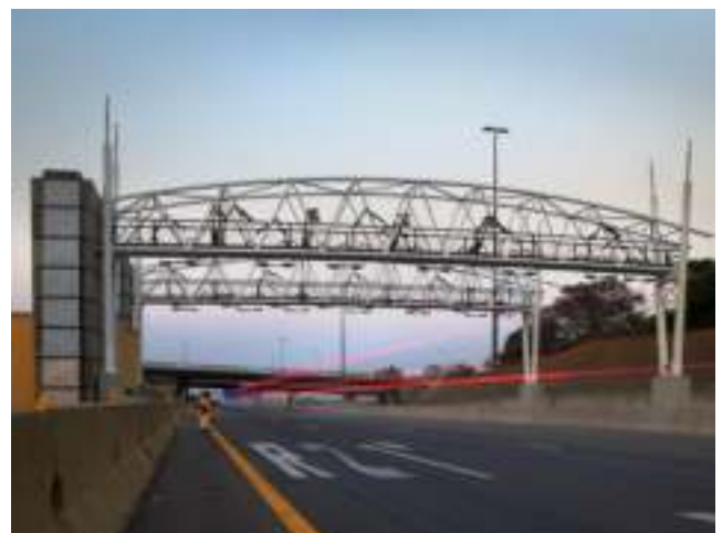
An example of a gantry in a multi-lane free flow system.
