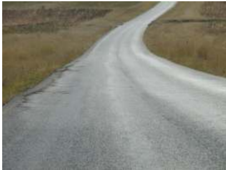
Figure 4-4: Example of a road with a 3.0 rating for its pavement adequacy.
