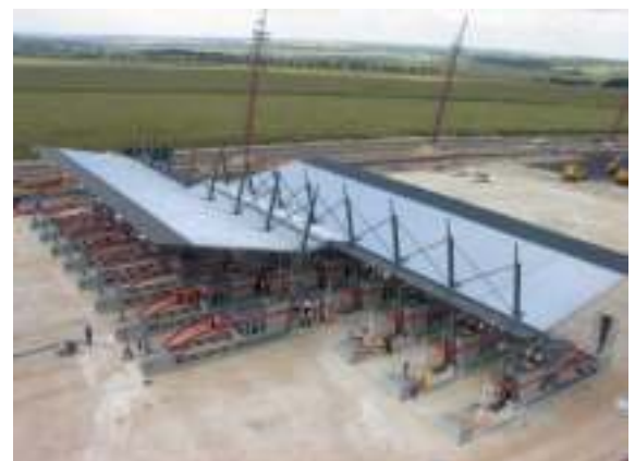
An example of a conventional toll plaza.
