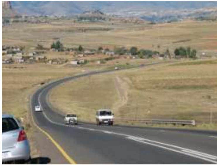
Figure 4-3: Example of a road rated 4.5 for its geometric adequacy
