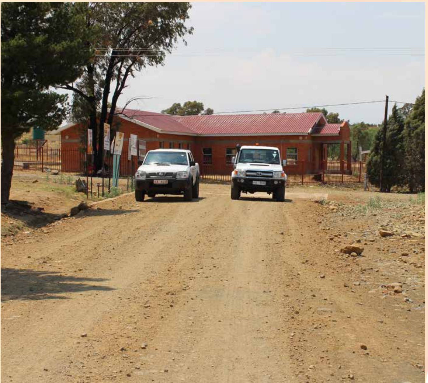
Maintenance of a Gravel road from Tsakholo to Litsoeneng sponsored by Road Fund
